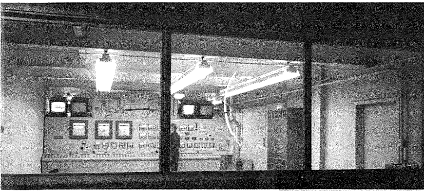
Rotary Kiln Control Room.
